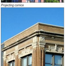
Parapet wall with projecting cornice
