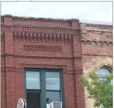
Parapet walls with projecting brick corbels
